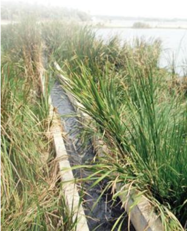
Sewage is let into the wetland for purification before reaching Jakkur Lake (in the backdrop)
